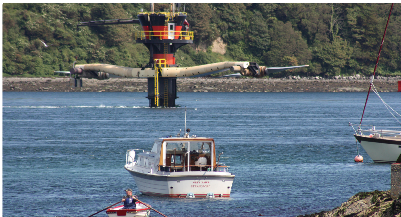
Figure 1. The SeaGen tidal turbine with its rotors withdrawn above sea-level
